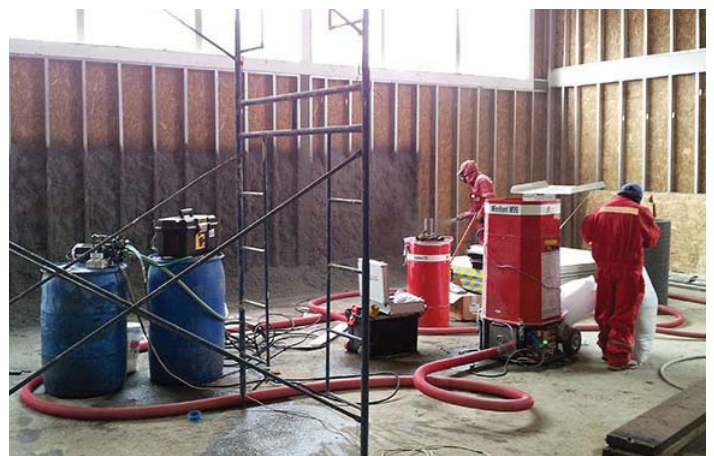
Chile: Damp spraying
