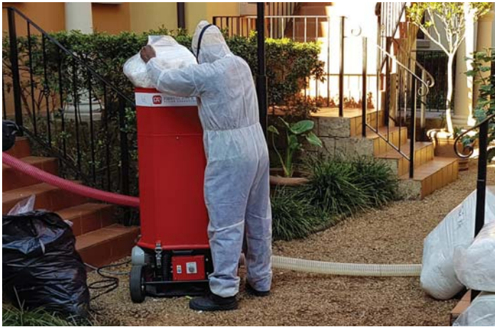
South Africa: Attic blowing with glass wool
