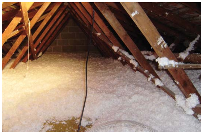
Attic blowing with glass fibre (NESTA SAS, France)
